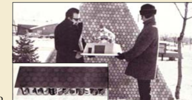
Left: R Sheldon (left) and H Hinterberger hold the model of the building to house the hydrogen bubble chamber at Batavia. The geodesic dome is to be constructed from triangular panels, as seen in the background, built of empty beverage cans (inset). Right: Some members of the buffalo herd at Batavia. (Photos NAL.)
