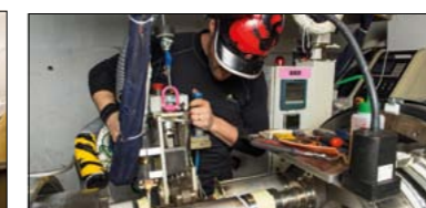
Left: Sporting the flags of Pakistan and France on his hard hat, a member of a SMACC team inspects a splice inside an opened “M-line” stainless-steel sleeve. On 6 February, the team opened the last M-line. Middle: Rebrazing the last LHC splice during LS1 on 10 March. Right: Members of the operations team – here Reyes Alemany Fernández, left – are joining in the work in the tunnel during LS1. (Image credits: left to right, Michael Struik/CERN, CERN-PHOTO-201403-045 – 04, CERN-PHOTO-201401-013 – 23.)
